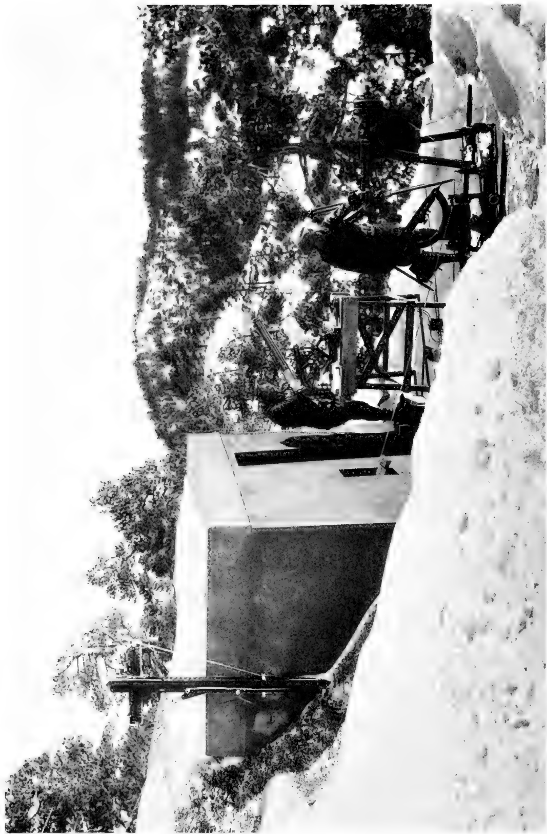
FIG. 1.—Table Mountain Solar Observatory. The bolometer which measures \frac{1}{1,000,000} degree temperature is in the tunnel, and sunlight is reflected into it.
